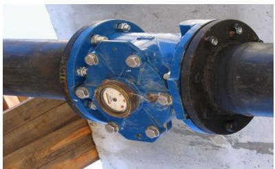
Figure 6.4 Measuring pumping rate by flow meter
