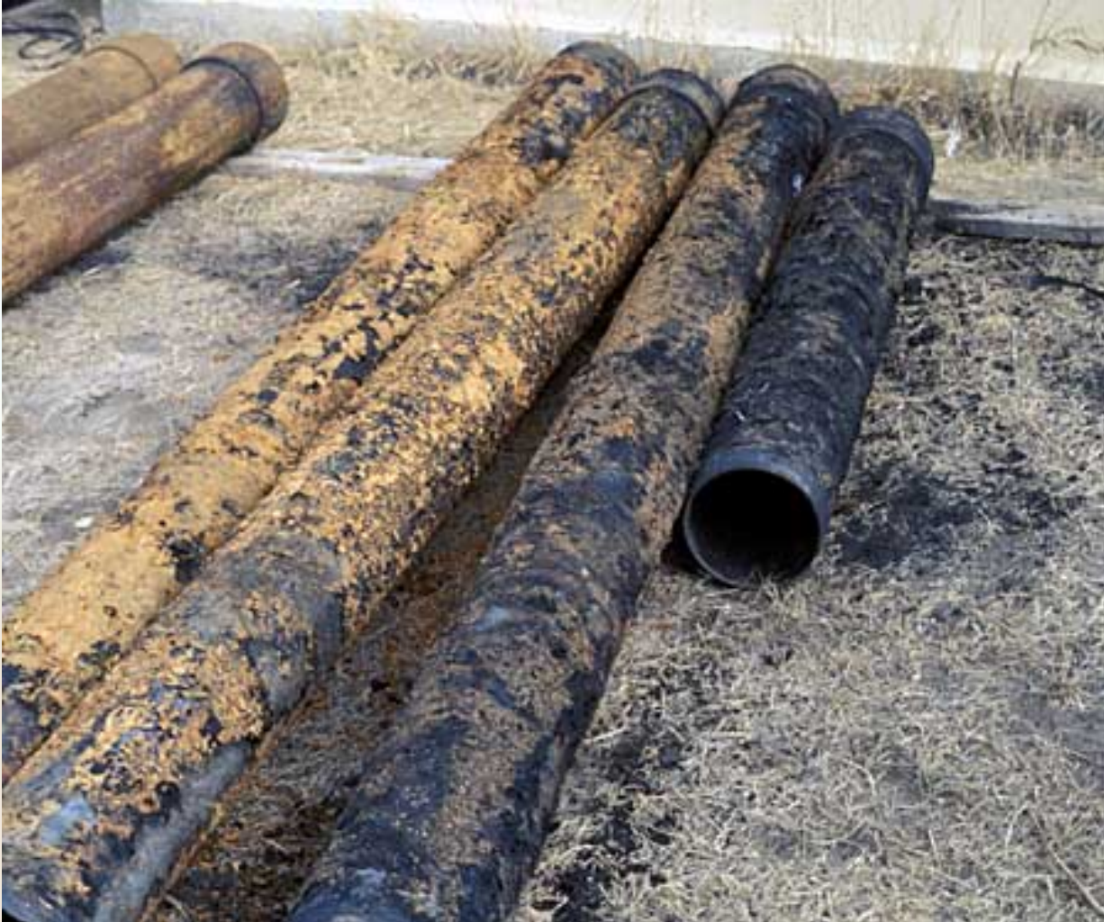
Figure 5: Iron bacteria on pump column riser pipe just removed from a well
