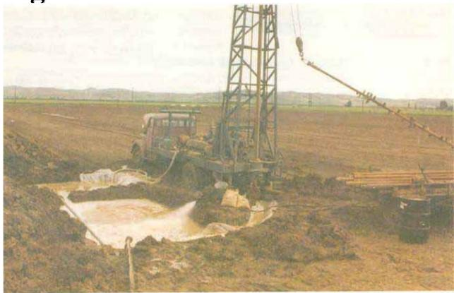
mud pump on the rig withdraws drilling fluid from this pit to inject down the drill rods to the bit. This Italian driller has lined the drilling fluid pits with polyethylene film to reduce fluid loss into the ground. Note the homemade hole cleaner or scratcher the driller uses to keep the borehole open during drilling.
